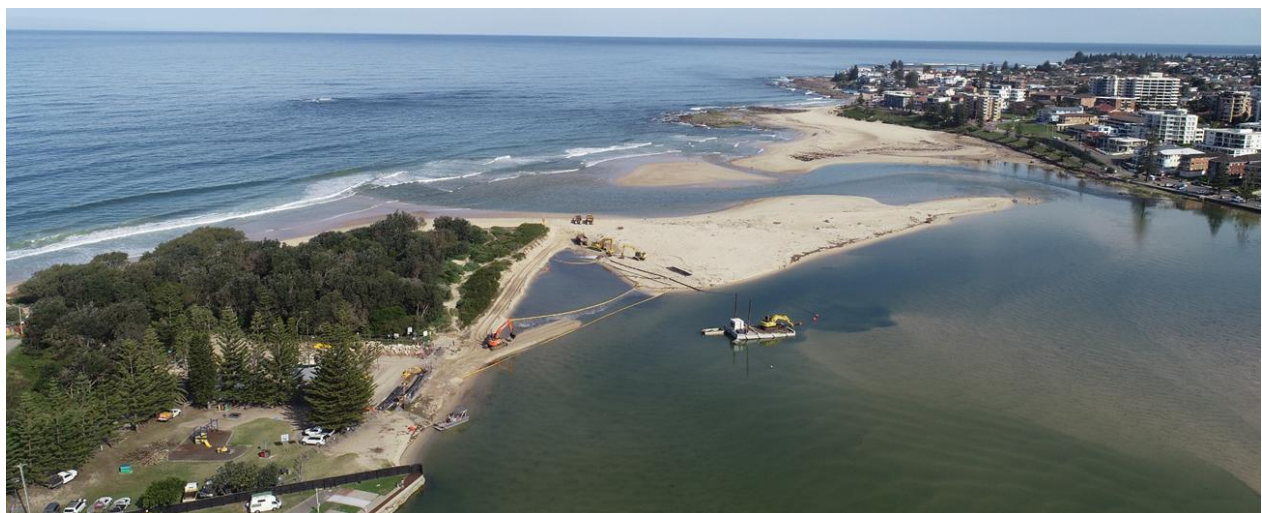
Figure 8: Photograph showing entrance dredging works in September 2020 (source: CCC).
