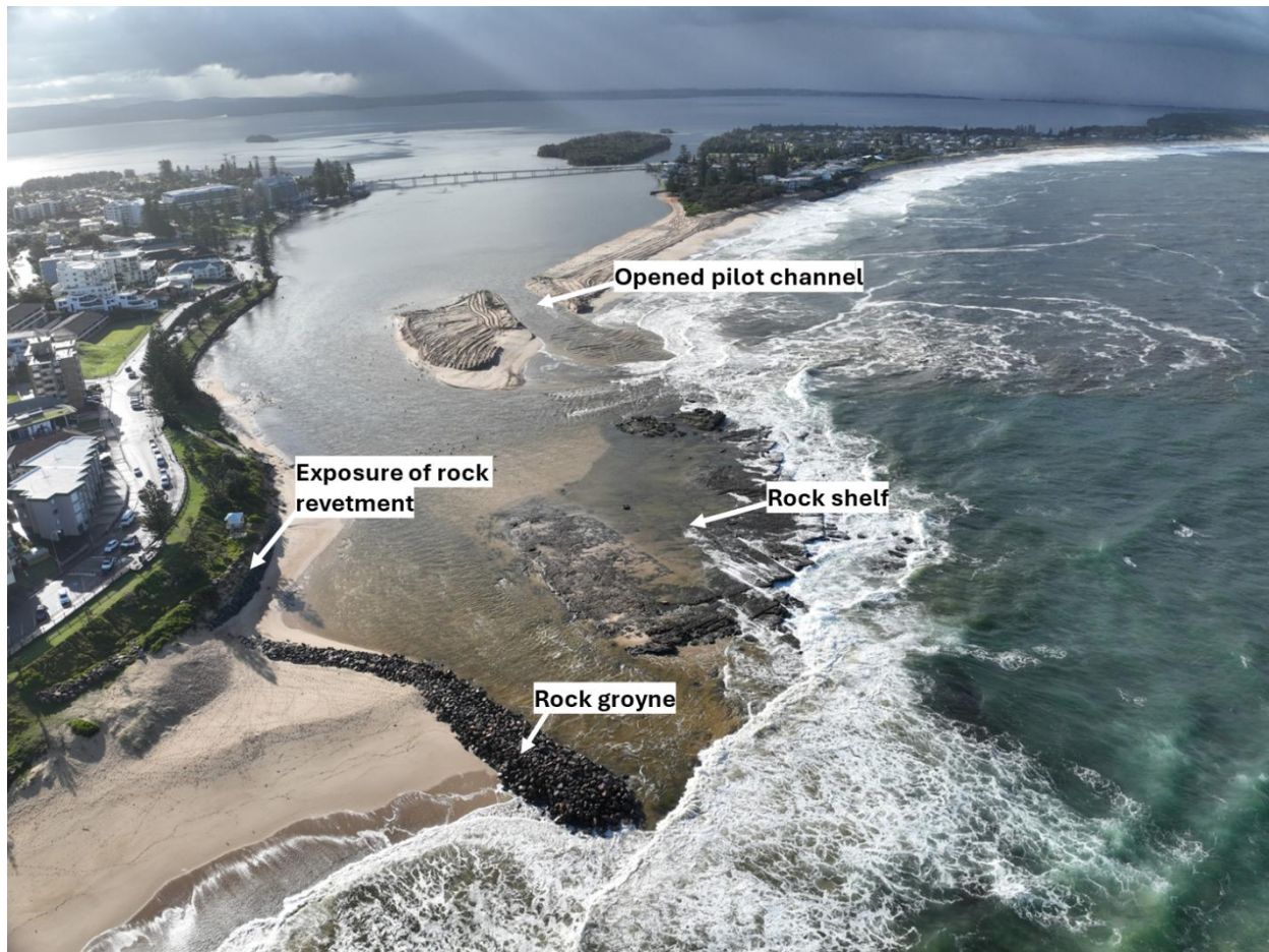
Figure 50: Photograph showing eroded area downdrift (north) of groyne and opened pilot channel in May 2025 (source: Chris Drummond/ DCCEEW).
